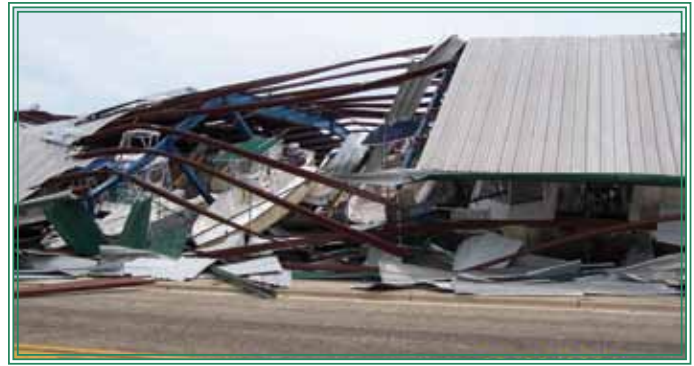
Older buildings have proven to be especially vulnerable. This one went over in Ivan.
