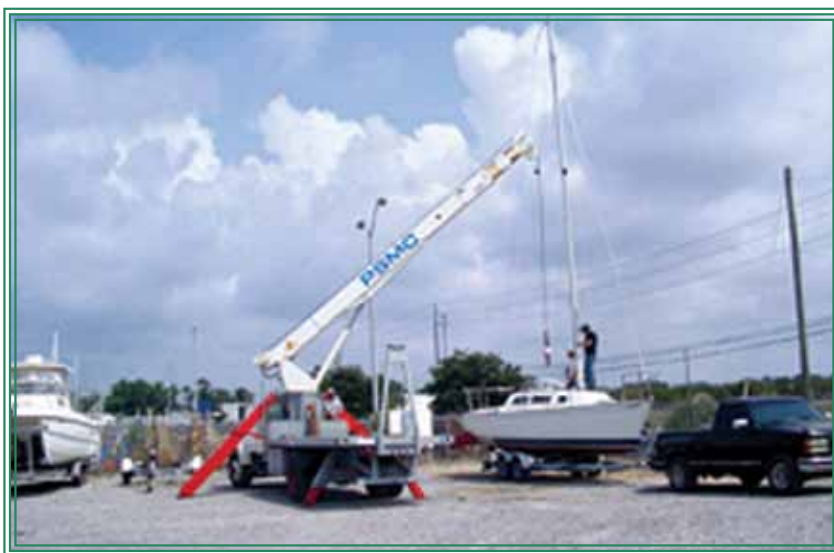
PSMC, Jacksonville, Florida: Using their portable crane, masts can be pulled fairly quickly—in as little as a half hour if the electrical wiring harnesses are disconnected and turnbuckles loosened.
